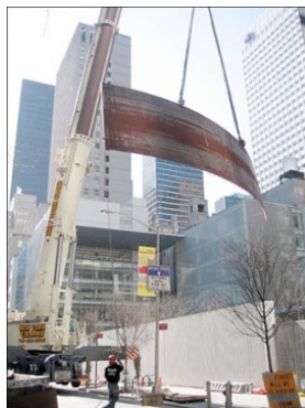
Richard Serra's Intersection VII being installed at MOMA
